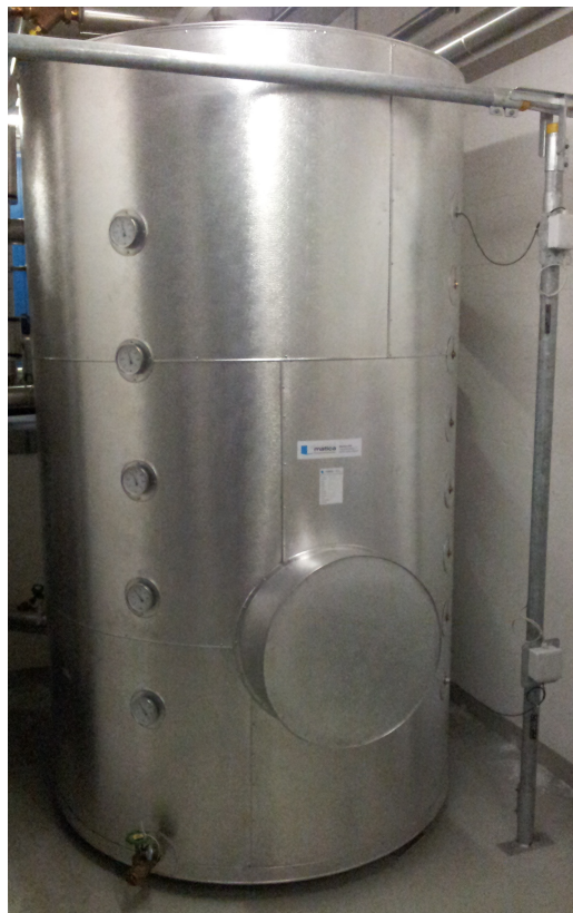
Fig. 3.6: Household hot water storage with reheated water
