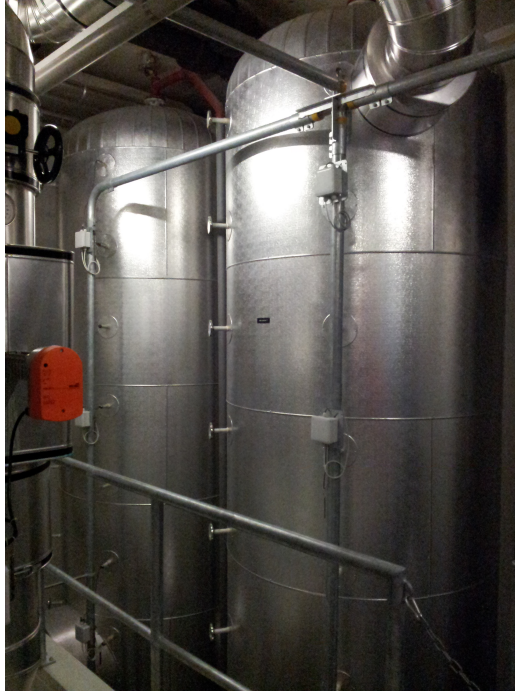
Fig. 3.3: Waste heat storages in the underground
