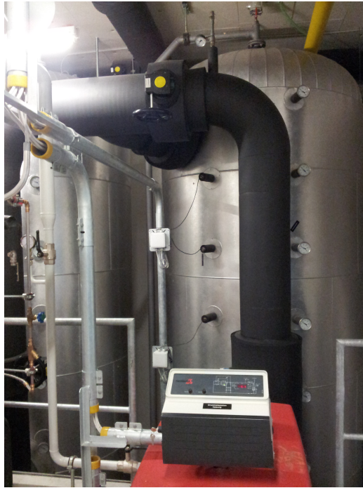
Fig. 3.2: Both cold water storages are located in the underground
