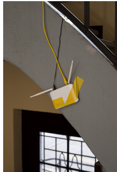
Figure 25: Additional WiFi Access Point to Cover the Basement
